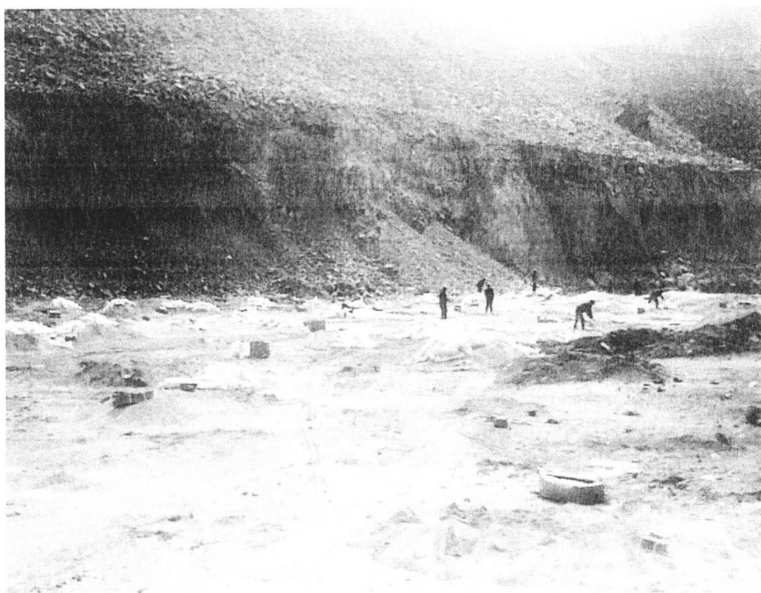
图 4.4 装药现场 Fig.4.4 The scene of blasting charge
